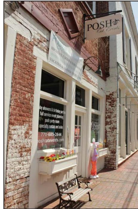
The vinyl banner placed directly above the transom window on this storefront is inappropriate because it is of incompatible material and obscures the façade.
